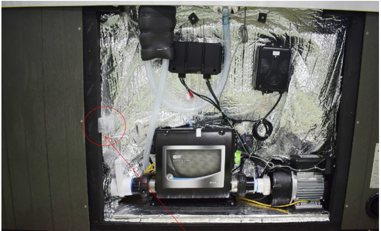
Jump wires position
