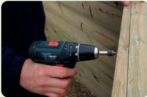
Fitting the Shelving Support
