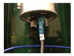
10. Connect red wire ('S' from soft start) to capacitor as shown.
