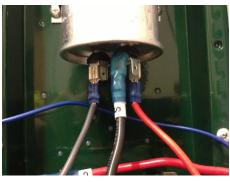
14. Connect all soft start wires as per wiring diagram
